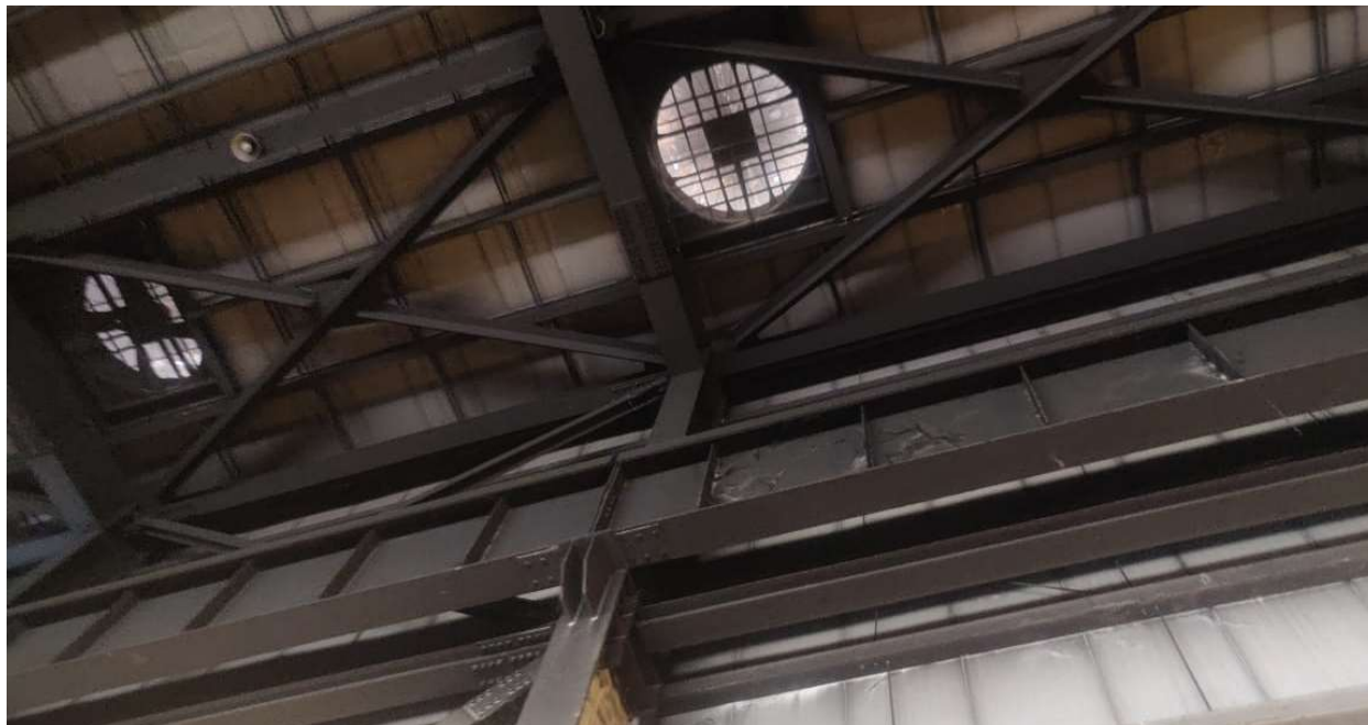
Figure-9 All Steel beams at Roof level are smoky due to fire incident and as well as the paint is deteriorated at various locations.
