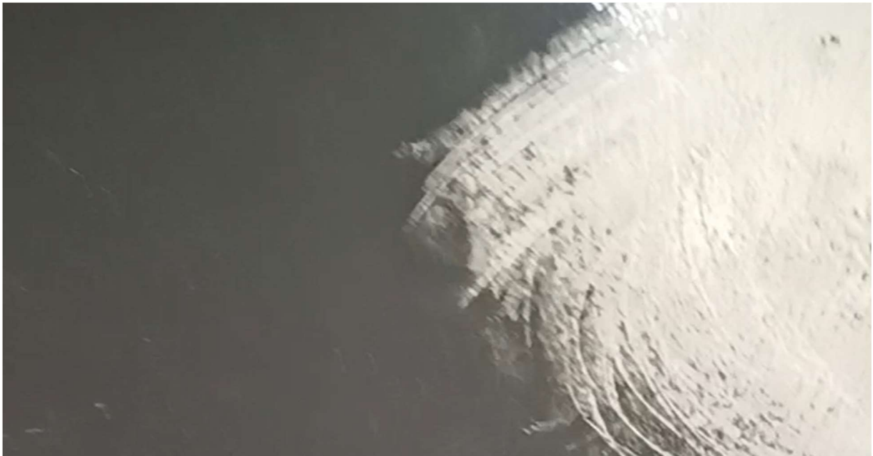
Figure-14 Smoke deposits from the steel beams were cleaned manually, and inherent color of steel beam can be seen.
